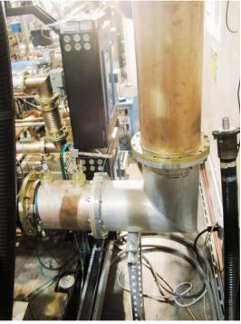
Coaxial cable (or hardline) is used for frequencies up to about 400 MHz and down to direct current, and waveguide at higher frequencies, where the loss is less than coax.
