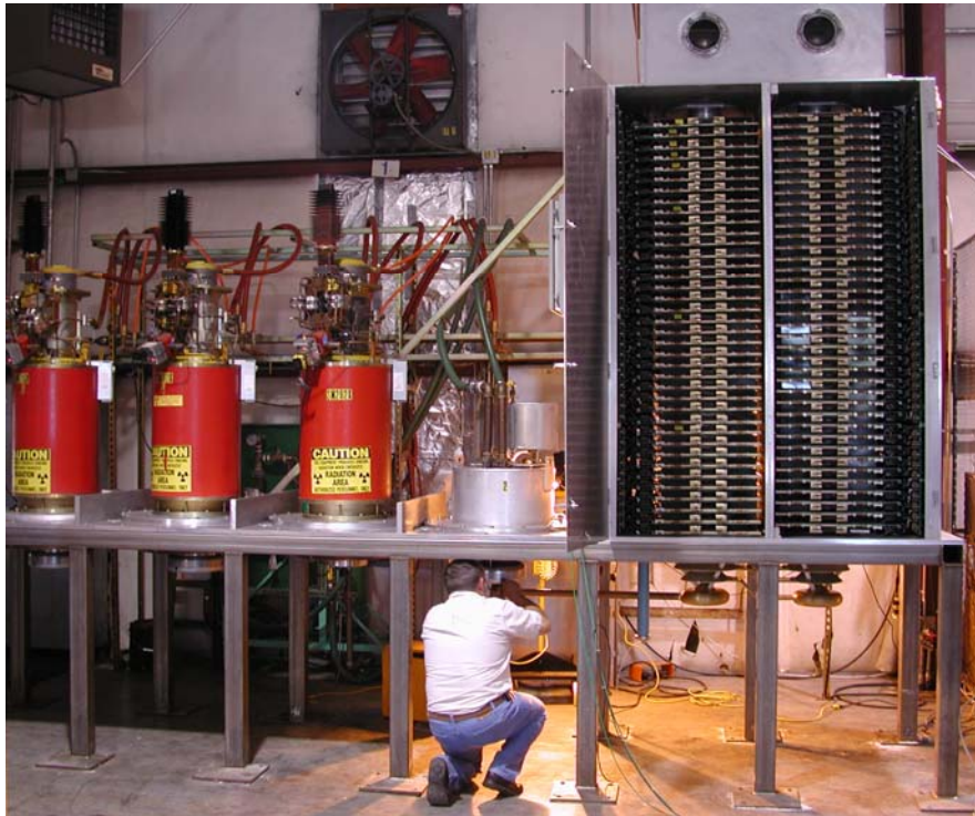
3 turn Secondary with water load
