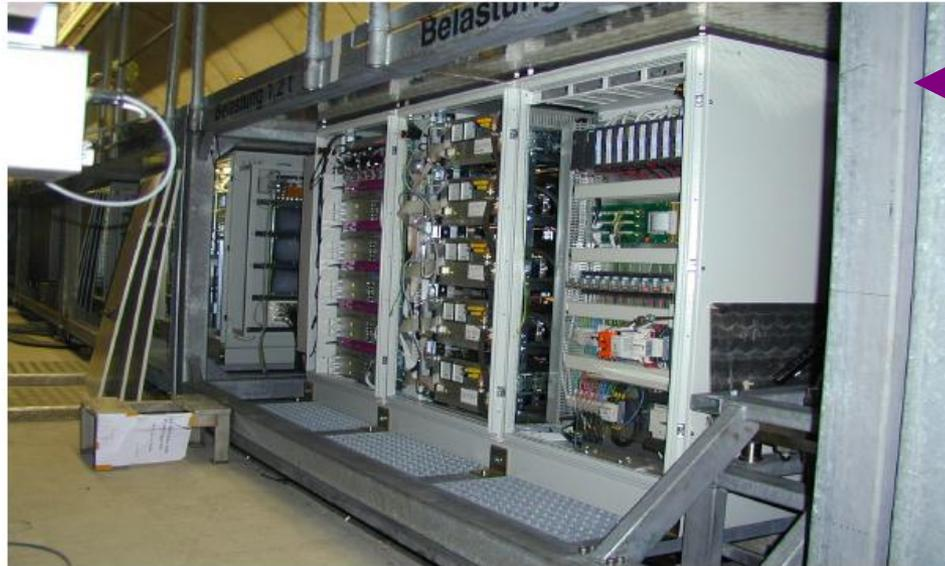
Power Supply Rack System with Docking → System for **fast replacement** of the entire unit
