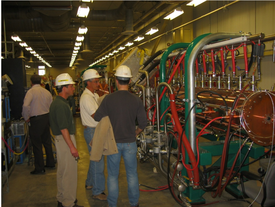
SNS DTL tanks 6 pre-install
