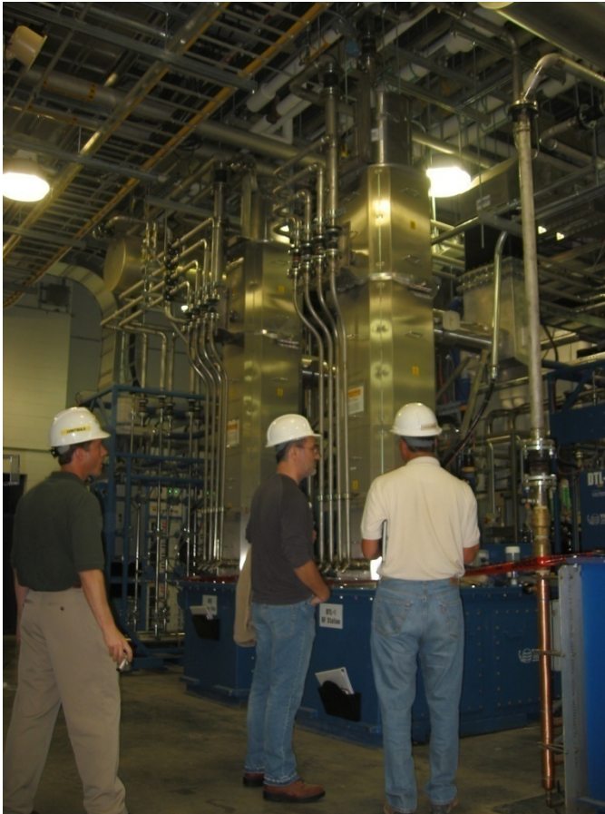
warm linac klystron galleries at SNS
