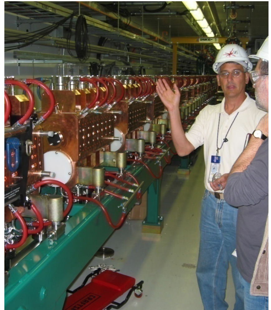
SNS CCDTL tanks installed in tunnel
