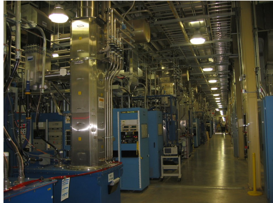
warm linac klystron galleries at SNS
