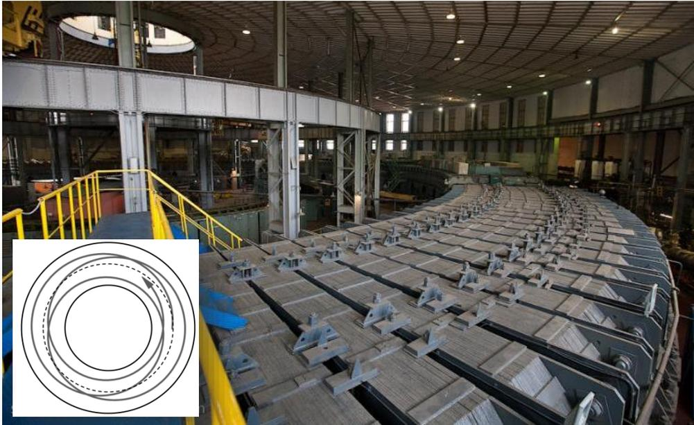
**10 GeV weak-focusing Synchrophasotron built in Dubna in 1957, the biggest and the most powerful for his time. It is ~60m diameter ring, and its magnets weigh 36,000 tons and it was registered in the Guinness Book of Records as the heaviest in the world.**
