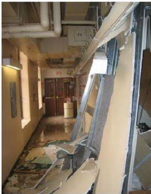
Figure 2 - Hallway Outside Laboratory Showing Explosion Damage
