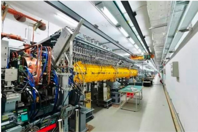
Figure 8: DTL-1 installed in the tunnel.
